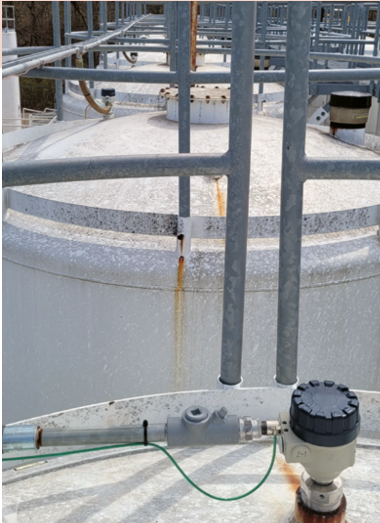
Level Measurement of Chemical Storage Tanks with NIVOTRACK Level Transmitters
