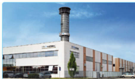
Production centre in Montagnana (PADUA), with the calibration tower in the background.
